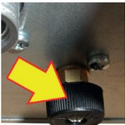
When the minimum pressure value is reached (0.6 bar), boiler operation is resumed.
