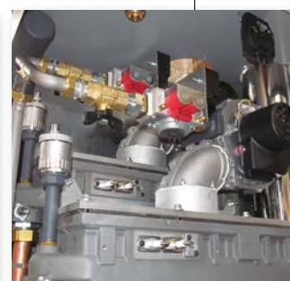
Group of: fan, modulating gas valve, premix burner
